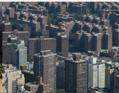
Illegal Construction Inspection
